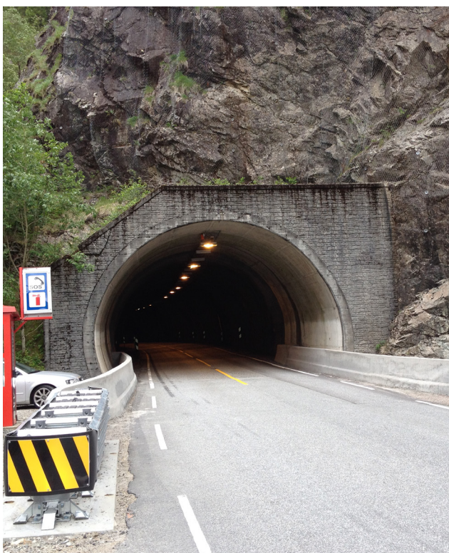
Giljajuvet tunnel | Foto: Tor Lomeland, Multiconsult
